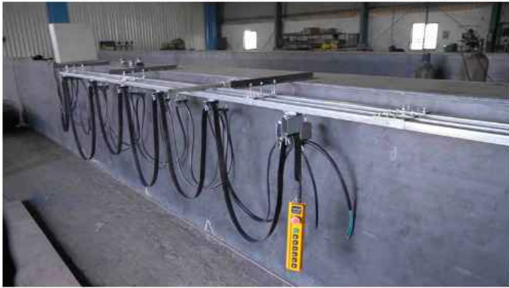
Anand C Rail Installation
