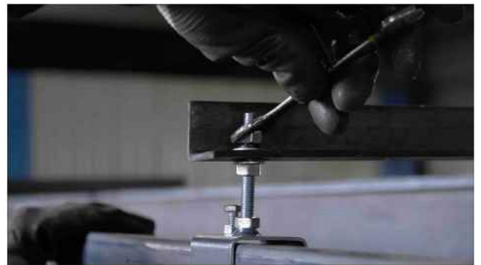
Anand C Rail Hangar Clamp Installation
