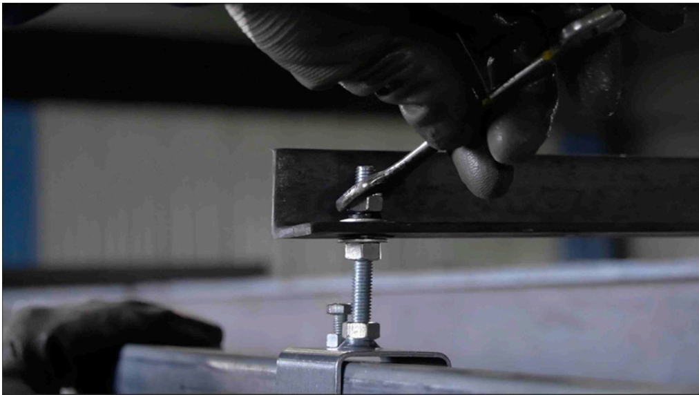
Anand C Rail Hanger Clamp Installation
