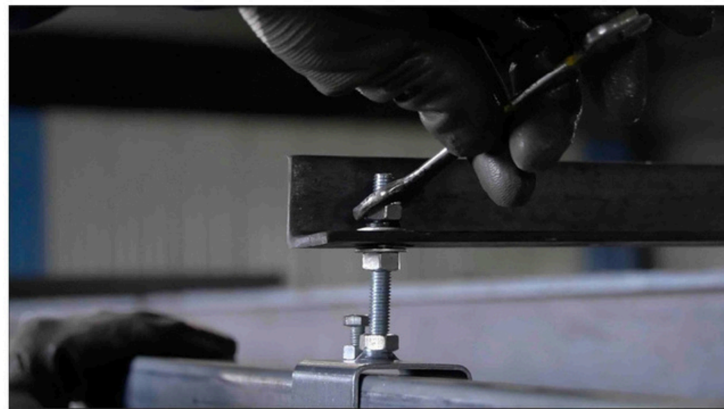
Anand C Rail Hangar Clamp Installation
